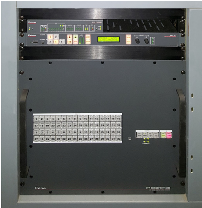
An Extron XTP CrossPoint 3200 modular matrix switcher in the control room provides AV and control signal switching and distribution within and between the Commander M. Neel Buell Lecture Hall, a second lecture hall, and Videoconferencing Suite 207.
